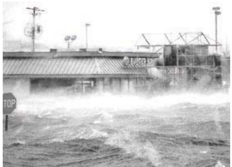
Water unleashed by Hurricane Katrina floods a Burger King restaurant in Moss Point, Mississippi. The Moss Point Social Security office is located just across the street.
